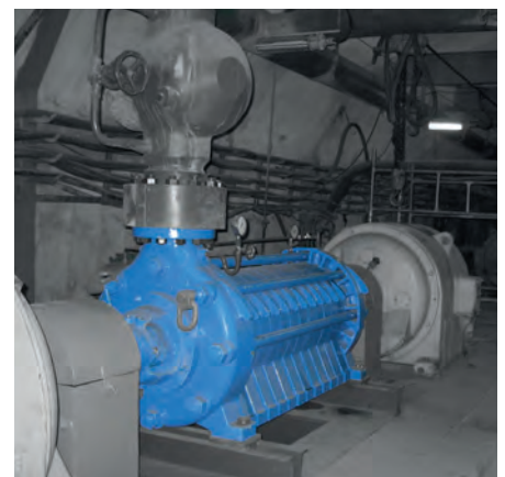
Intermediate flange at stage casing
